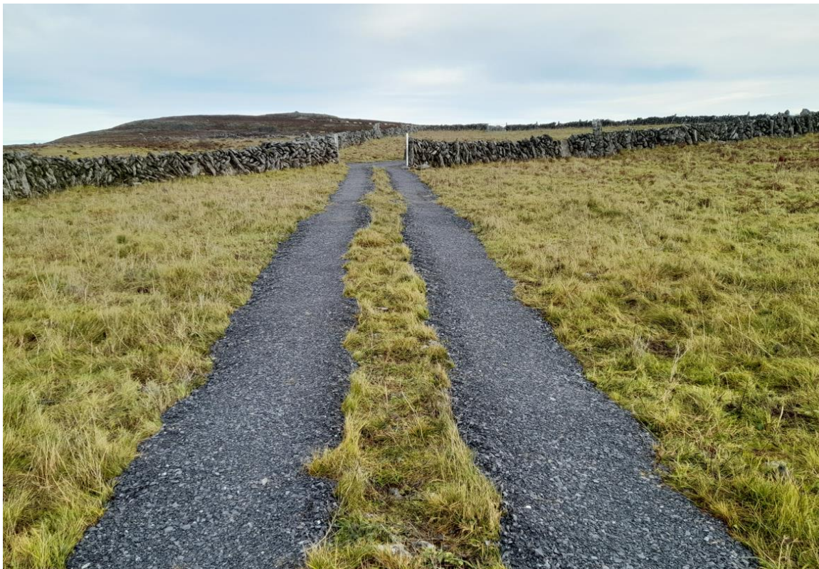
Picture 12: Example of Track Re-surfacing Gravel
