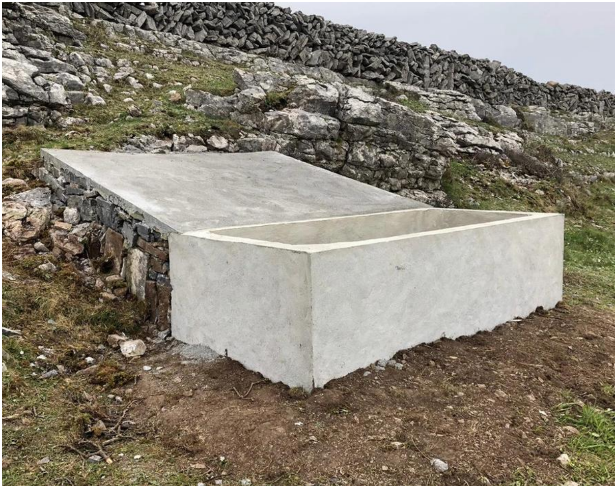
Picture 9: Example of a Rainwater Catcher
